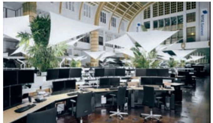
Fabric on Supporting Tensile Structure
